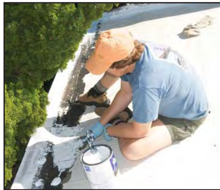
The Roof Project: More than 20 members volunteered over three days, to work on power washing, scraping and gutter cleaning, crack and window caulking, painting two coats of roof material, and a super clean-up, lead by head project manager Byron Jacobs.
