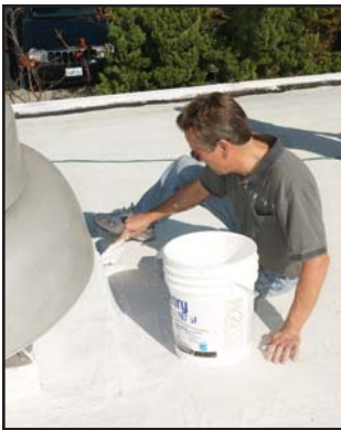
The Roof Project: More than 20 members volunteered over three days, to work on power washing, scraping and gutter cleaning, crack and window caulking, painting two coats of roof material, and a super clean-up, lead by head project manager Byron Jacobs.
