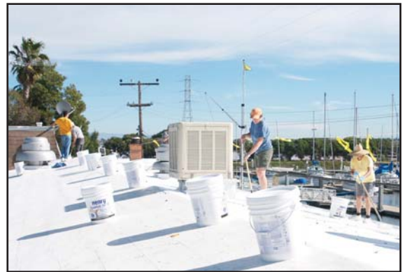
The Roof Project: More than 20 members volunteered over three days, to work on power washing, scraping and gutter cleaning, crack and window caulking, painting two coats of roof material, and a super clean-up, lead by head project manager Byron Jacobs.
