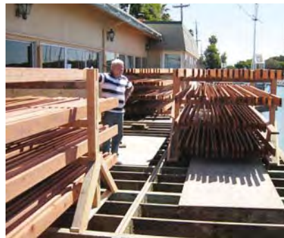
Deck Project: Beefed up supports, deck boards drying, Mark and Tim Peterson conferring.
